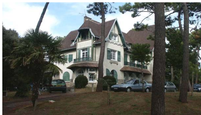
Bridge Club - Avenue H. de Balzac
